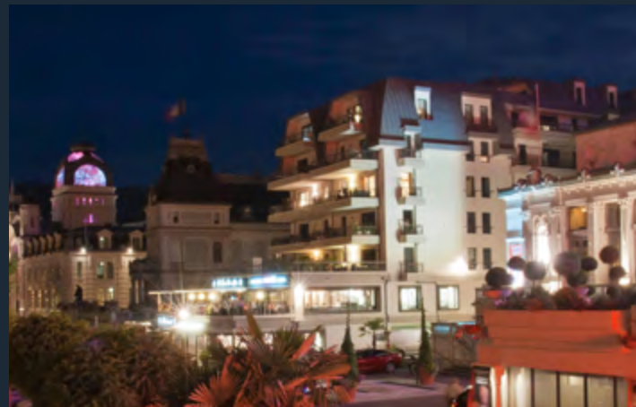
La Coupole Evian-Les-Bains
